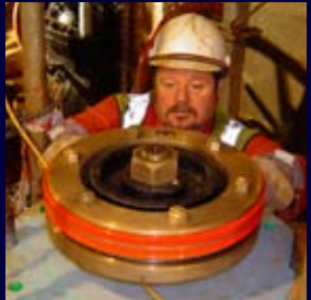
Valve refurbishment Derbyshire
