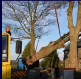
Storm damage Longridge
