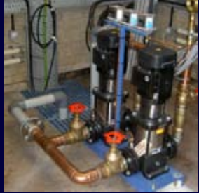
Supply and installation of pumping equipment
